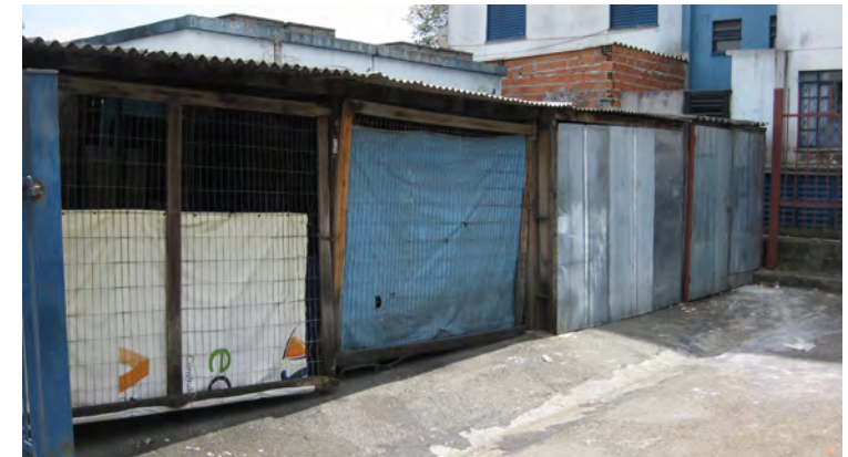
Self-constructed garages to provide secure car parking in Gleba A
