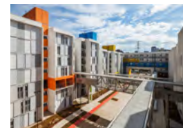
4. Gleba G, 420 units, completed 2013
